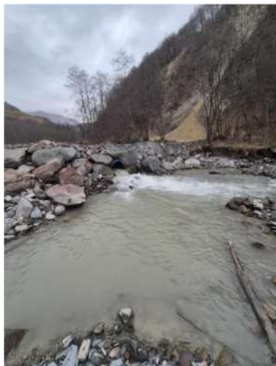
Figure 2.4. Placement area of bridge (N 3), third fishing point.
