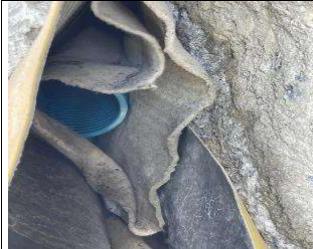
Tunnel water arrangement at tunnel after completion of linings lot-2
