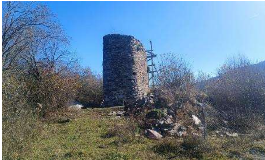
Figure 23: Conservation Works of Didveli Backed Tower (CH Site #10)
