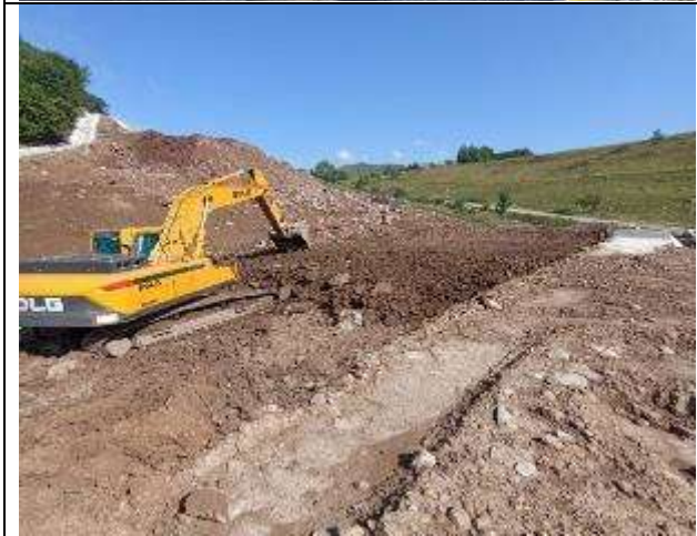
Ongoing Construction activities at Gudauri Access road project September 2024
