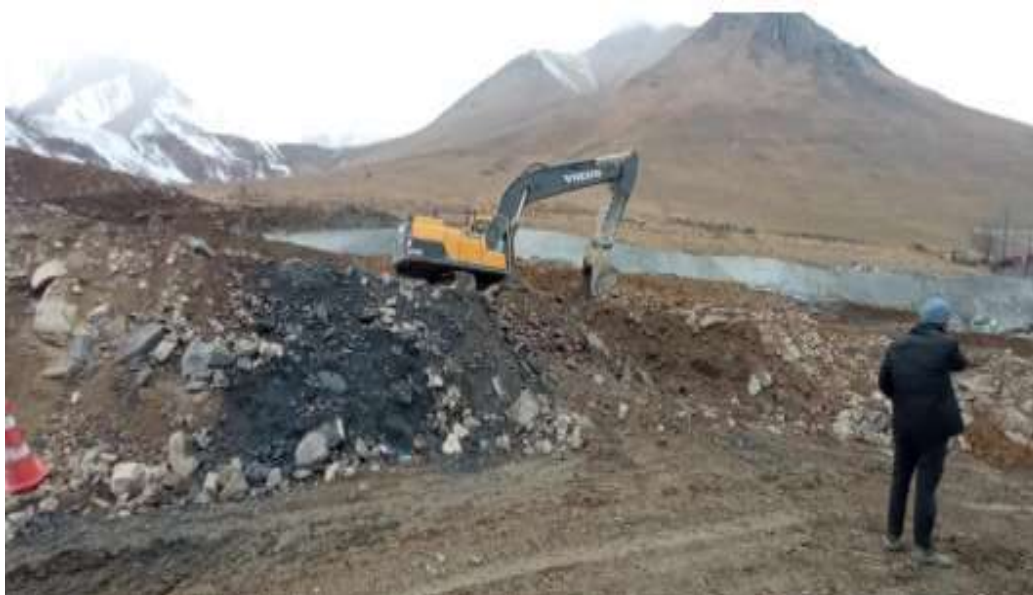
Figure 38: Access arranged to Cemetery by Contractor for Lot 1
