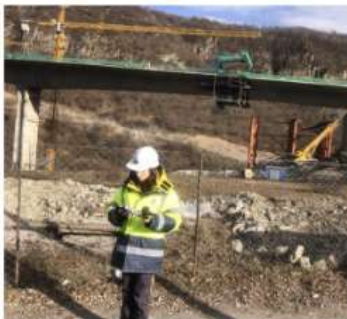
Figure 5.2.1 Noise (NM#2) Monitoring Point – Around the Bridge #2
