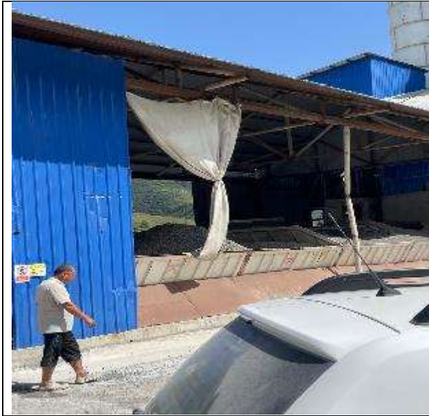
Material covered for the use in batching plant 1 September 2024
