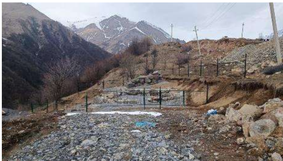
Figure 24: Relocation Completed for CH #26
