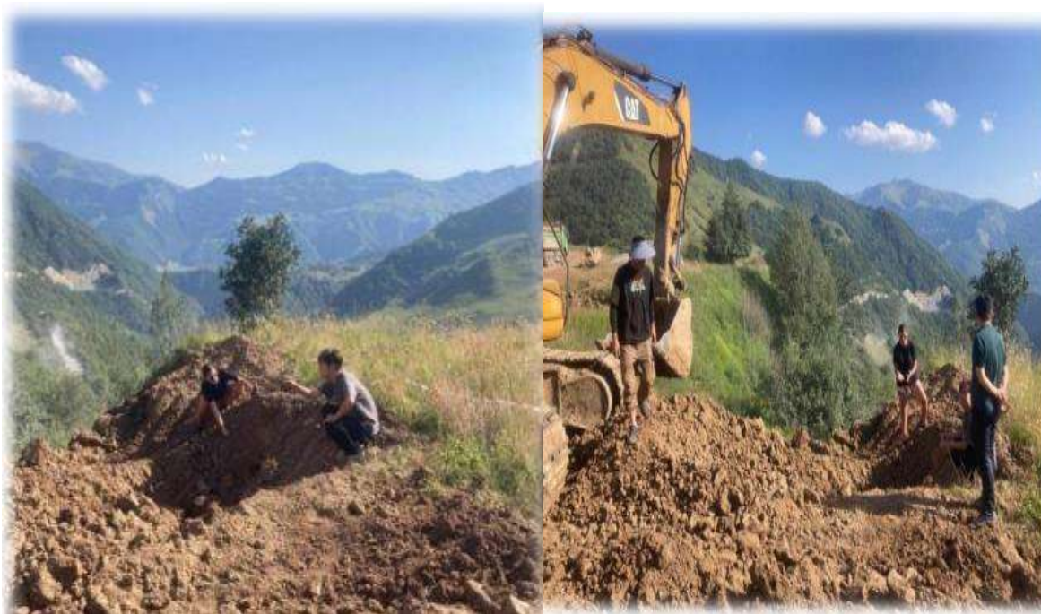
Figure 33: Onsite Training for Topsoil stripping in Benian-Begoni Village (August 2024)
