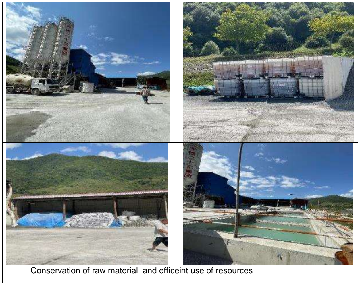
Figure 39: Best Practices adopted by Contractor at Lot 2
